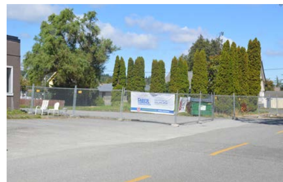
CONSTRUCTING THE TALMON — Construction fencing went up Aug. 15 at the 306 Center Street site for the 3-story 19-unit residential building. — Photo by Ken Stern
