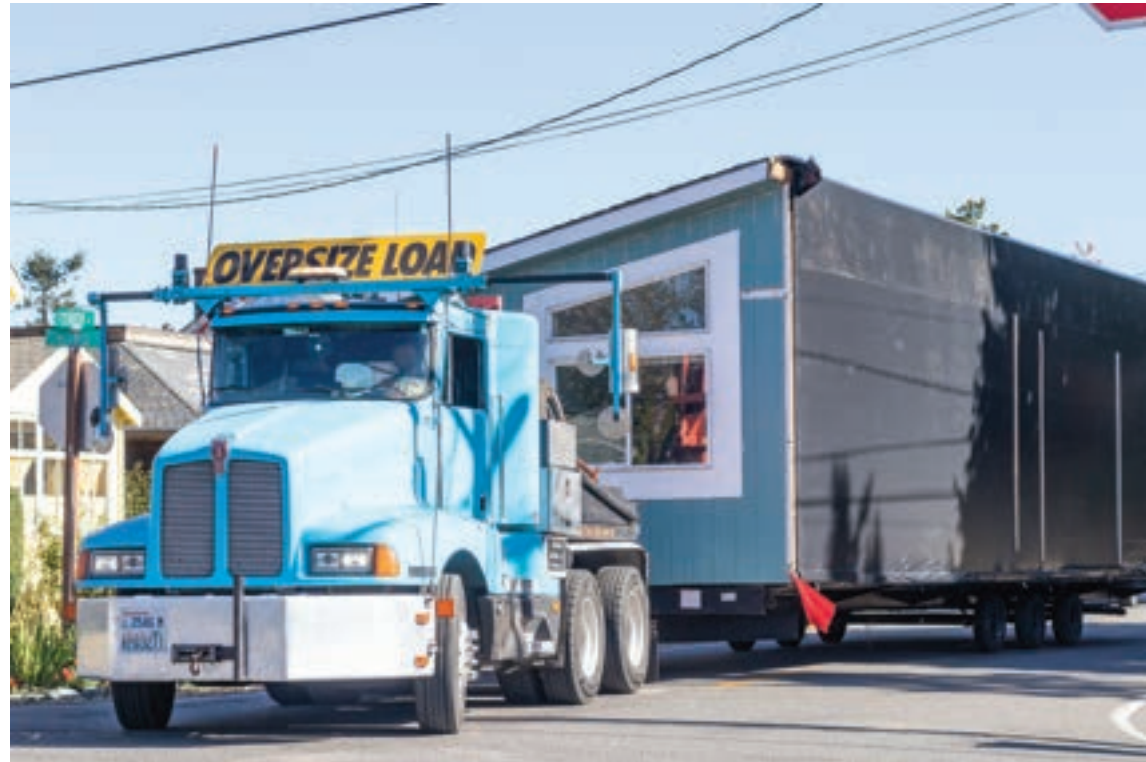
MAKING ROOM FOR BUILDING ON CENTER STREET – This double wide mobile home was removed from its Center Street site east of North Third Street Oct. 11 as the property owners prepare for building a 21-unit condominium building at Center and Fourth streets. – Photo by Marissa Conklin
