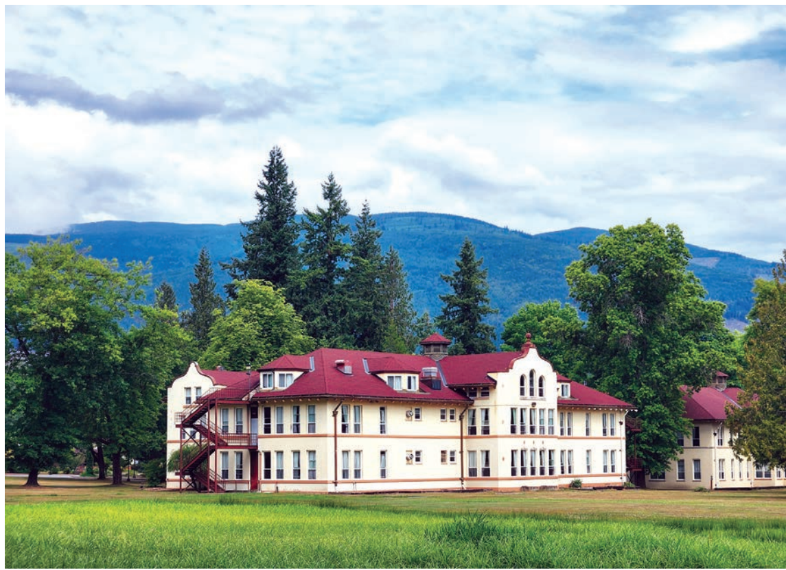
SPANISH REVIVAL — Most of the buildings on the Northern State Hospital campus feature Spanish Revival architecture. Some buildings, such as this one, have been maintained. Many other buildings have sustained vandalism and weather damage since the facility closed in 1973.
