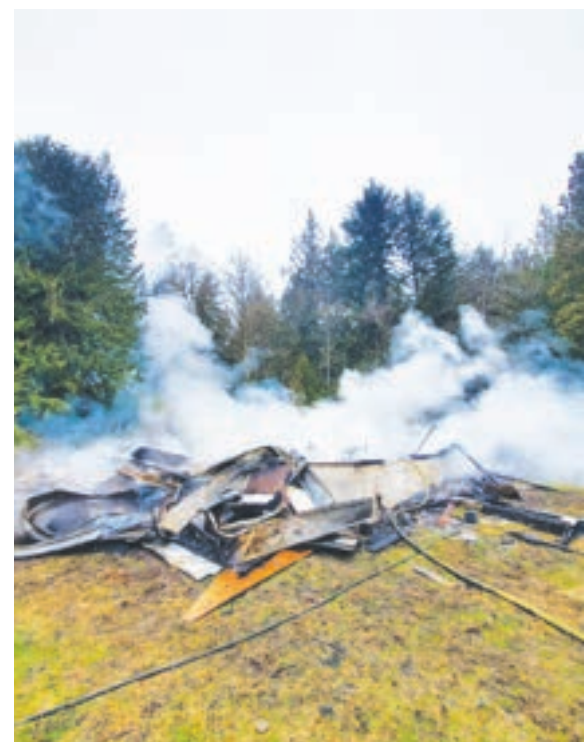
BURNING QUESTIONS – Authorities are probing the cause of a fire last Tuesday that leveled the house that Tyrone McLeod was building off Indian Road. Neither he nor his children were at the structure when the blaze started. A fundraising effort has begun to help recoup the family's losses. – Photo courtesy of Linda Rumbolt
